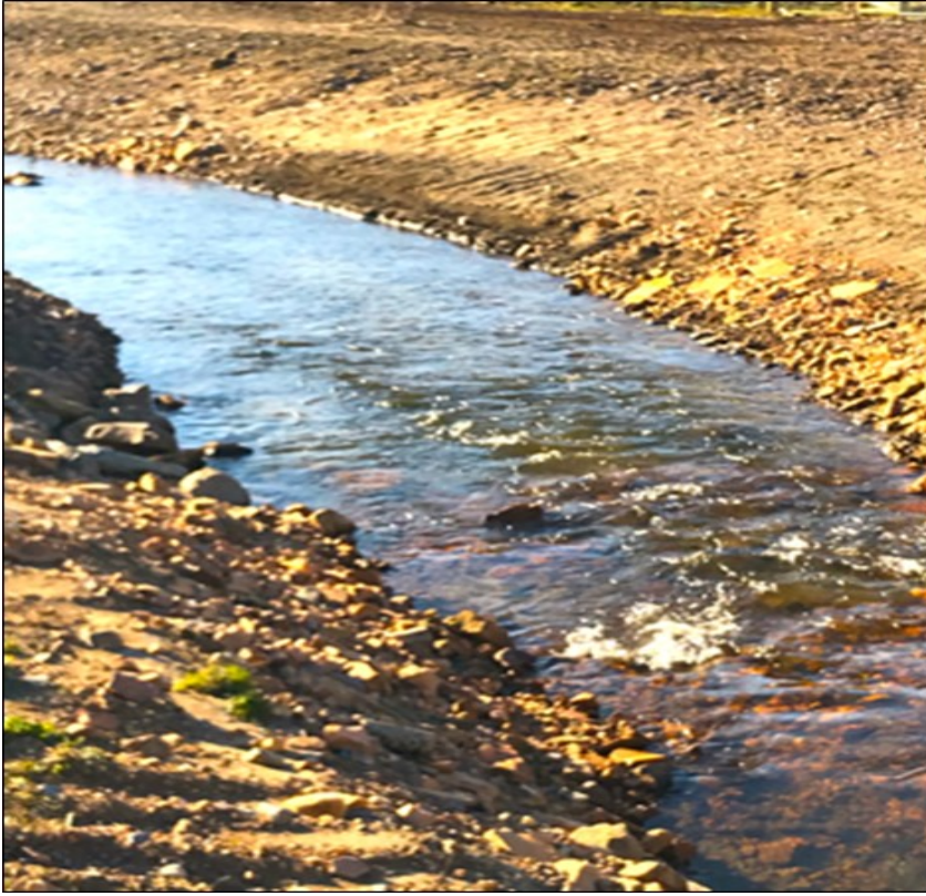
Figure 7. Much of the new part of the Beltie Burn, of the River Dee, below a new bridge, is shallow, and contains a great deal of silt and stones, washed in from the new banks.
